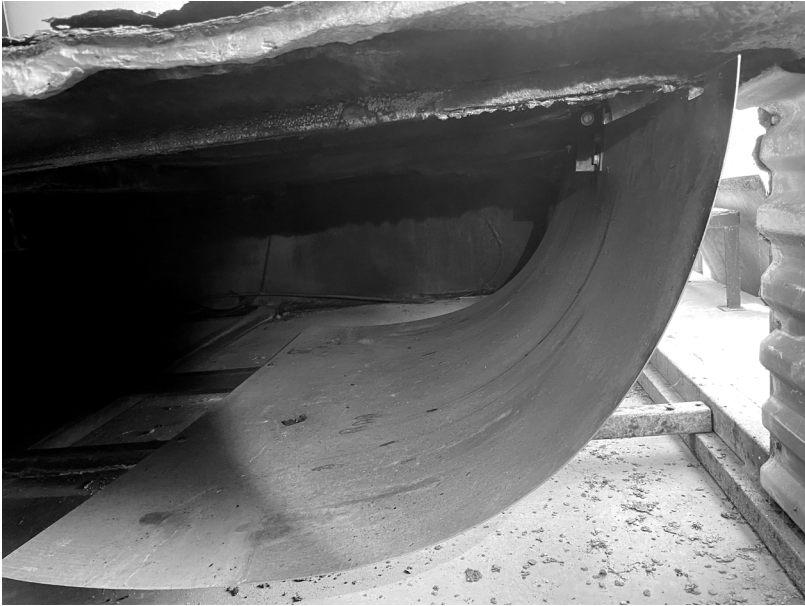
Figure 10-1. Sheet metal turning vane added to the lower-air plenum to improve airflow.
