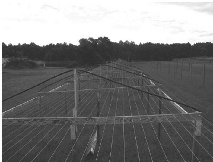
Figure 14-5. High-tensile-wire curing structure.
